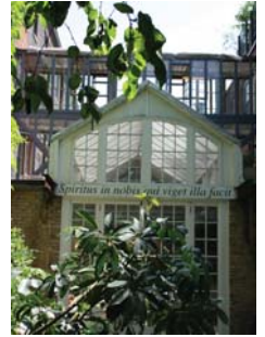
Courtyard view of bridge
