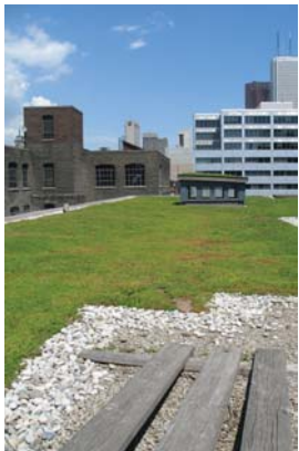
Extensive roof garden
